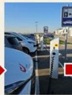
Electric charging station
